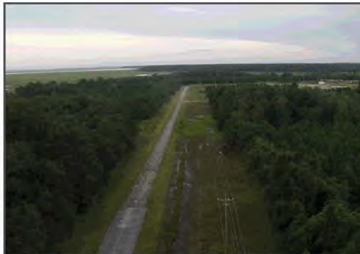
F-Existing power lines and road corridor
