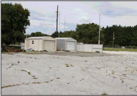
A-Existing structures near proposed main gate location
