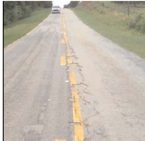
PAVED STREET WITH CRACKING
