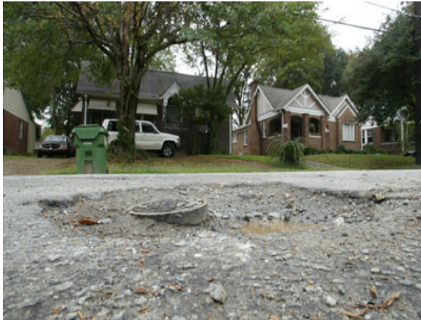
PAVED STREET WITH WATER DAMAGE
